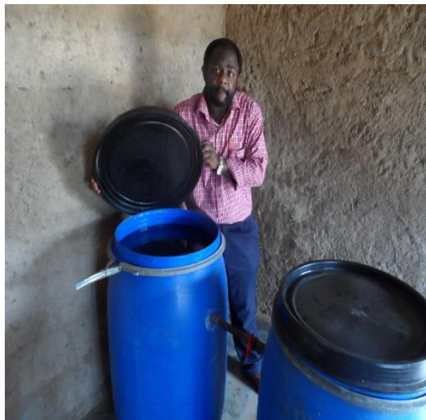
Figure 3 Sand filter drum Drum 1 (left) – sand filter media Drum 2 (right) – collection /storage of filtered water
